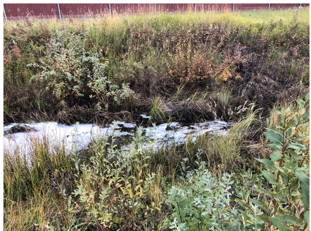
Photo 6: AFFF-water in ditch. View downstream towards culvert.
