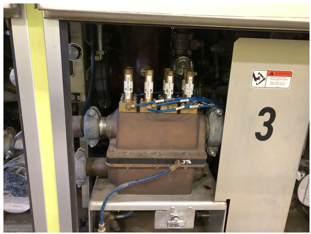
Photo 4: Engine Plate Style AFFF Proportioner
